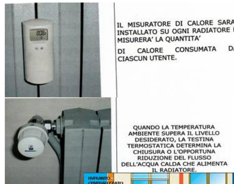
IL MISURATORE DI CALORE SARA' INSTALLATO SU OGNI RADIATORE E MISURERA' LA QUANTITA' DI CALORE CONSUMATA DA CIASCUN UTENTE.
